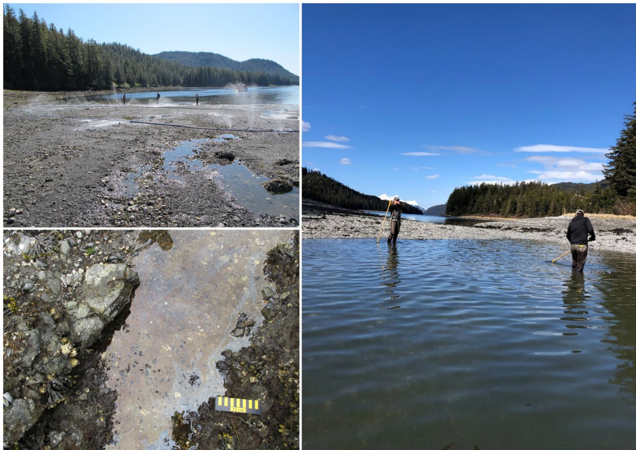
Figure 4: Examples of shoreline observations and treatment provided by the SCAT team: High-volume, low-pressure seawater deluge (top left), oil on beach near grounding sit in May 2022 (bottom left), shoreline manual agitation (right).
