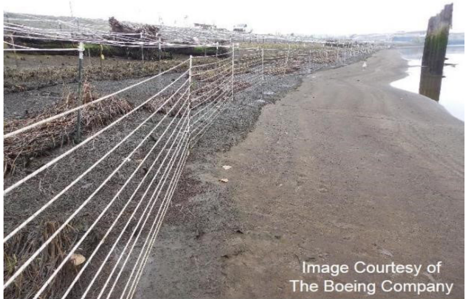
Figure 43: Goose exclusion fencing used initially at the Boeing project. This initial design did not work well; extensive grazing of marsh vegetation by geese occurred despite the fencing.
