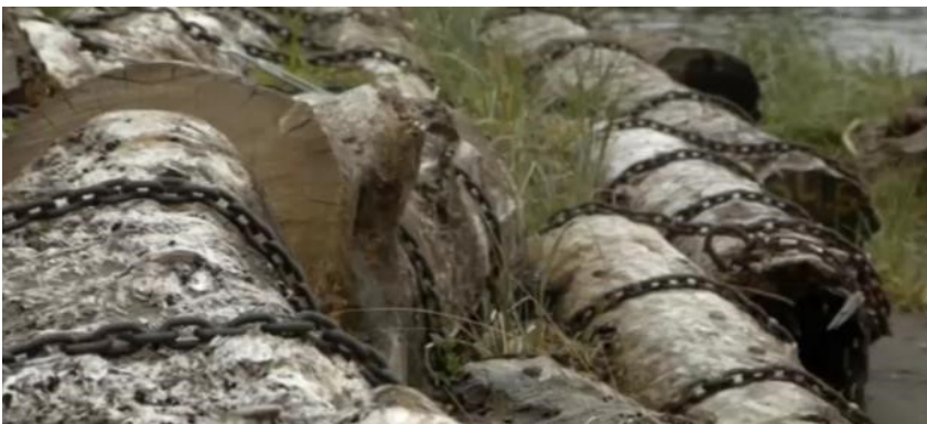
Figure 33: Close-up view of log placement showing anchoring chains. (Courtesy of the Port of Seattle)
