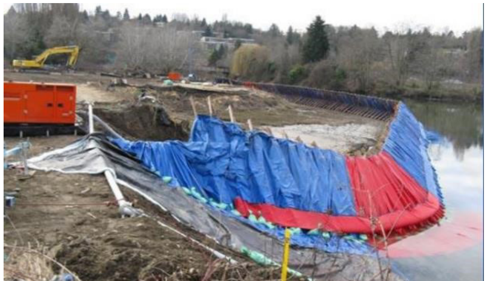
Figure 44: Site isolation and water intrusion at North Winds Weir site. (Photo courtesy of King County Department of Natural Resources and Parks)
