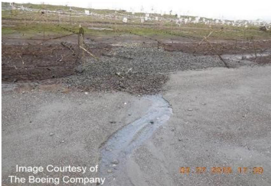
Figure 50: View (from the riverside looking inland) of groundwater seep area covered by gravel.
