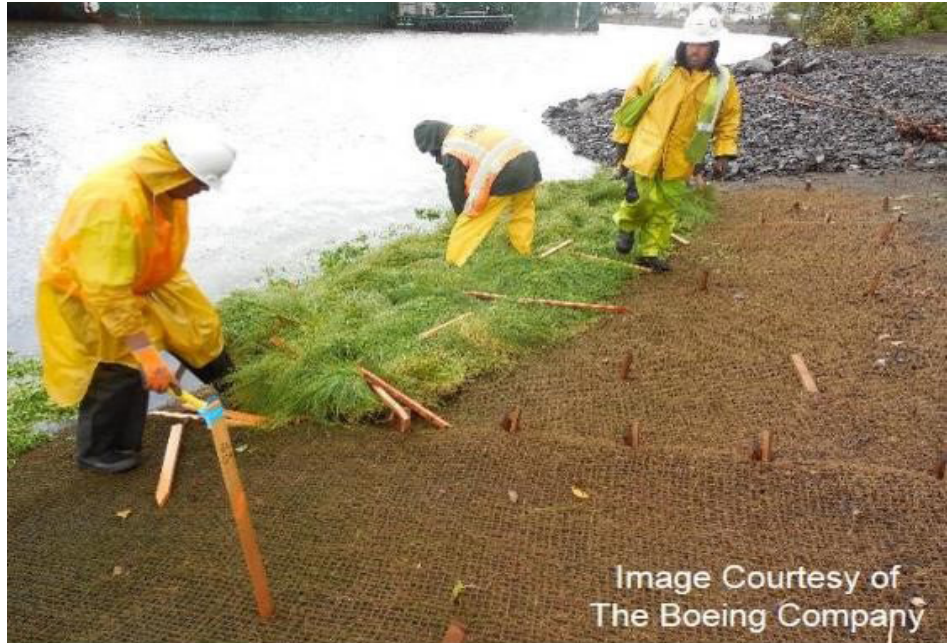
Figure 40: Installation of pre-vegetated coir mats in the marsh zone at the Boeing project.
