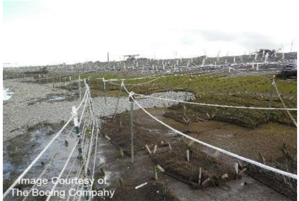
Figure 49: Alongshore view of patches of gravel placed at groundwater seeps at the Boeing habitat project.
