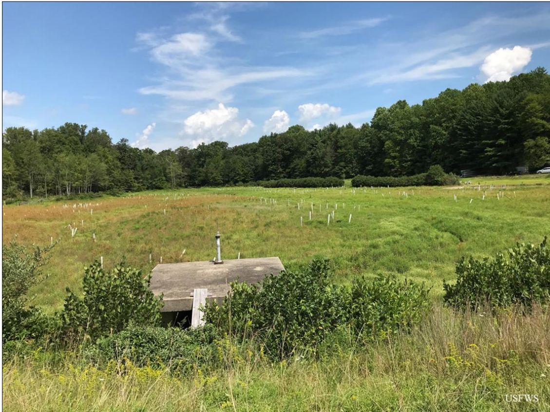
Figure 18. Beisler Lake in fall of 2019. The impoundment was permanently drained through the outflow structure embedded in the earthen dam in 2017, and the impoundment was partially revegetated in 2018.
