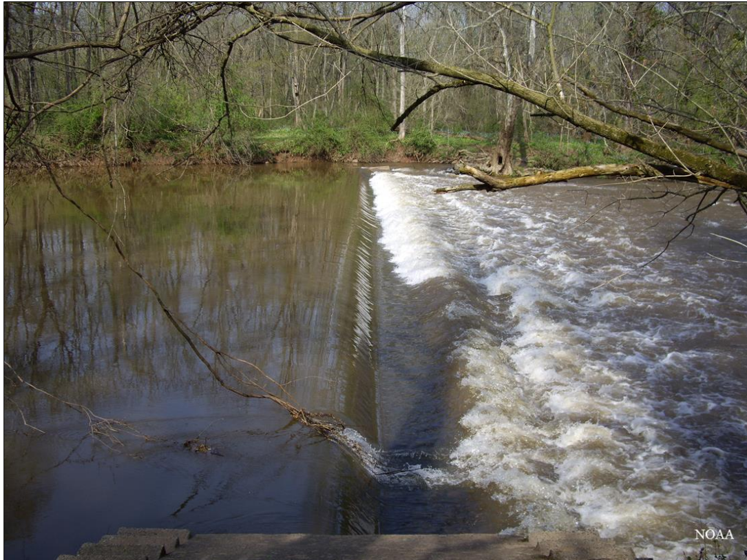
Figure 19. Mill Street Dam shown facing northeast. Water has eroded the stream bank along the northeastern edge of the dam, and visibly flows around the weir.
