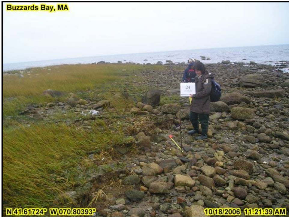
FIGURE H-2. Eroding Marsh Peat Scarp and Monitoring Stake and Photostation #24
