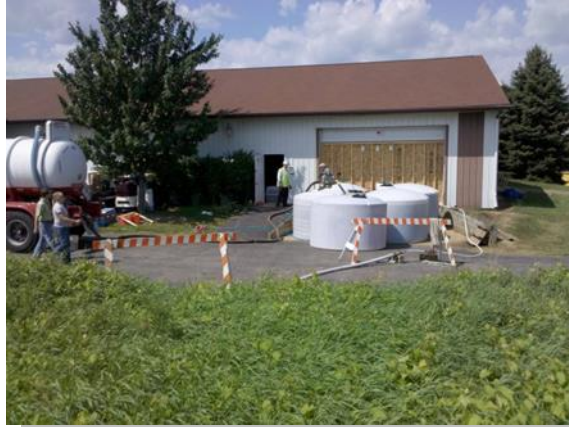
Wastewater tanks and vacuum truck
