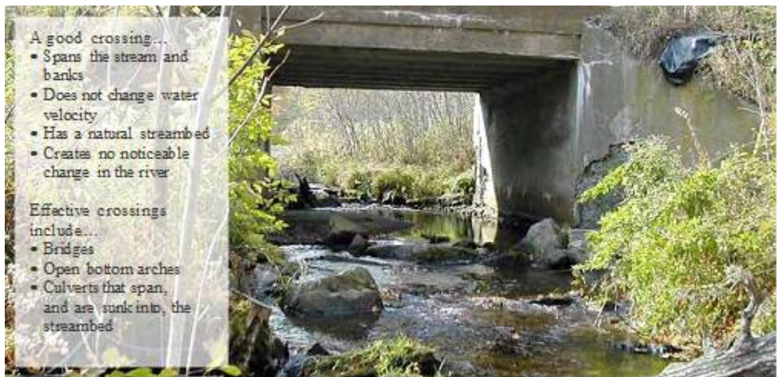
Figure 4.3. Example of an open bottom structure, along with general guidance for road stream crossings (Massachusetts Department of Fish and Game, 2005)
