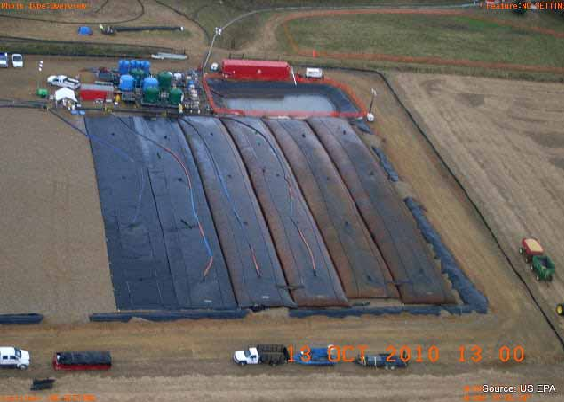
Geotube filter system used to capture contaminated sediment.
