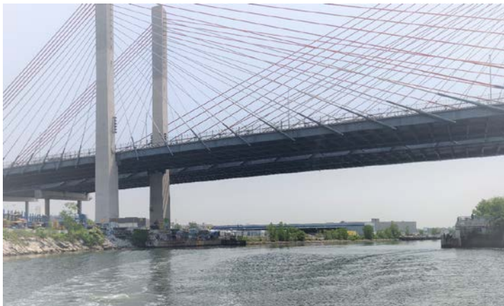
Kosciuszko Bridge over Newtown Creek.
