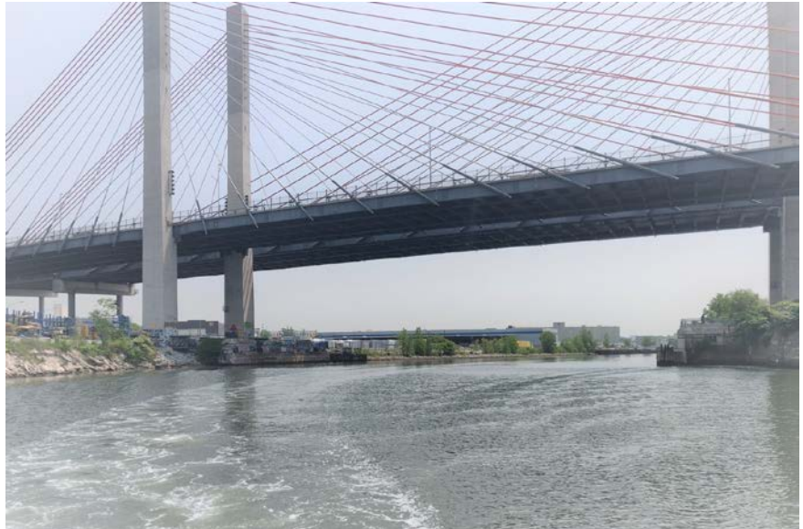
Kosciuszko Bridge over Newtown Creek.
