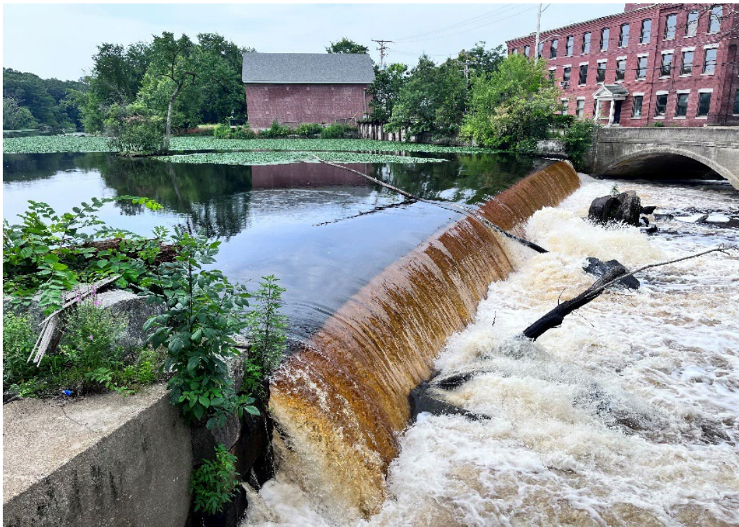
Figure 4. Talbot Mills Dam in 2022 (photo by USFWS).
