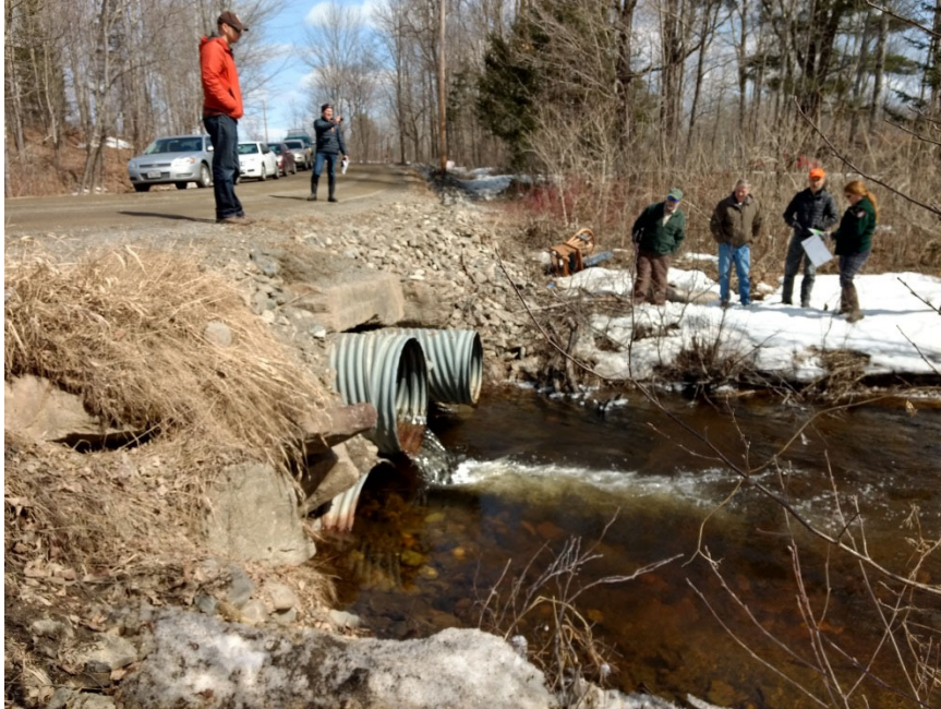
Figure 6. Perched and undersized culvert proposed for replacement at the crossing of Bacon Rd. over an unnamed tributary of Crooked Brook
