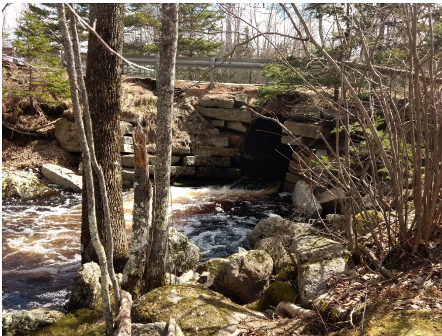
Figure 5. Perched culvert at Rte. 15 crossing over Snow Brook in Sedgwick.
