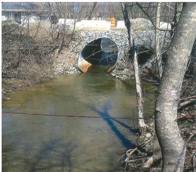
Figure 7. Undersized culvert on Sucker Brook on Lane Construction property.
