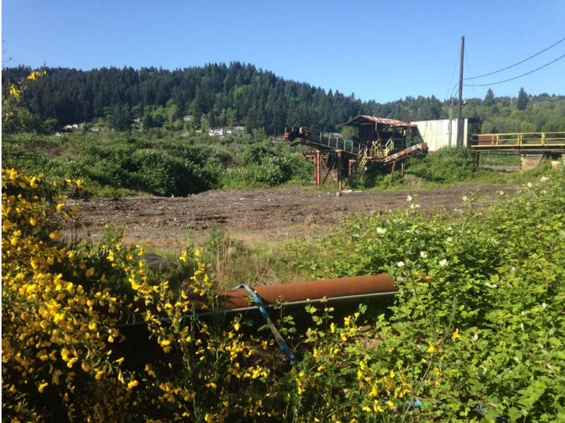
Photo Point 6 SW-facing (May 3, 2013 – pre-construction)
