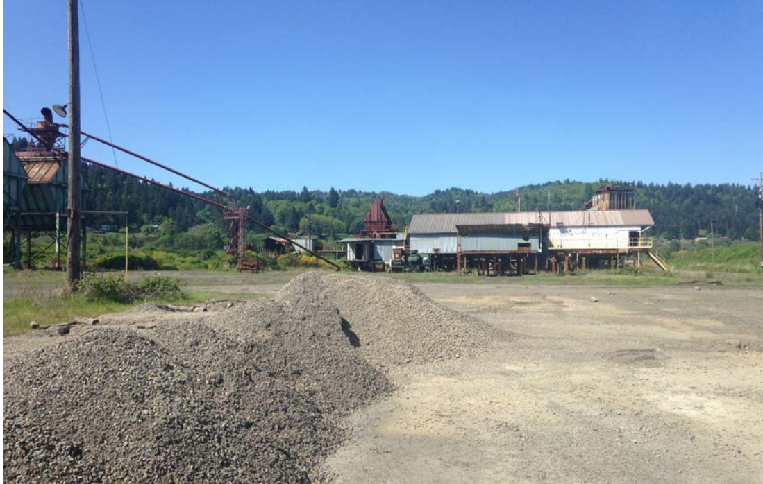
Photo Point 8 West-facing (May 3, 2013 – pre-construction)
