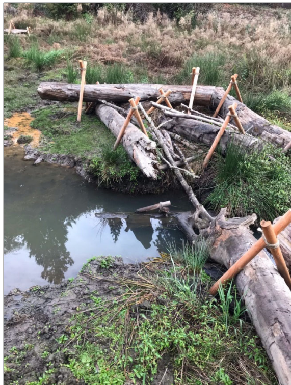
Figure 6 Log structures with completed maintenance showing new “ties” and crossing vertical logs brightly colored and freshly purchased. The new vertical members were installed by hand to avoid impacts to the wetland.
