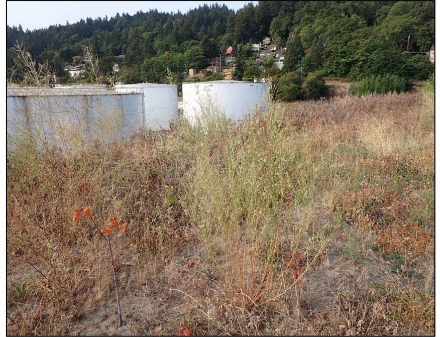
View looking south.
