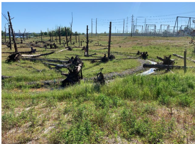
August 8, 2021 – photo facing east
