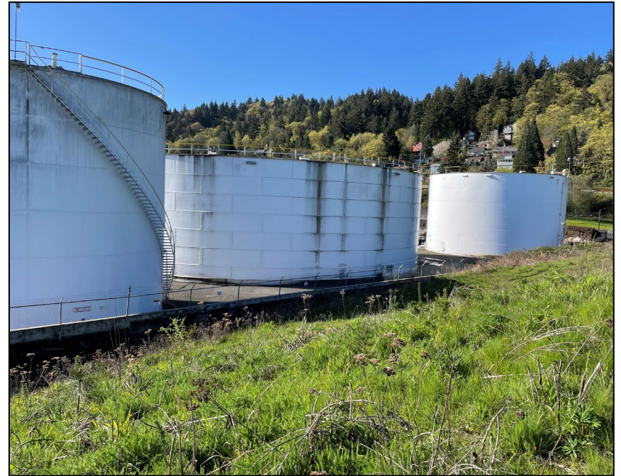
View looking south.
