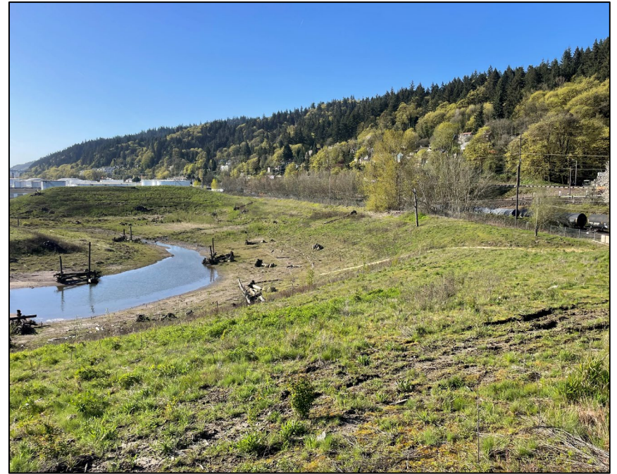
View looking south.
