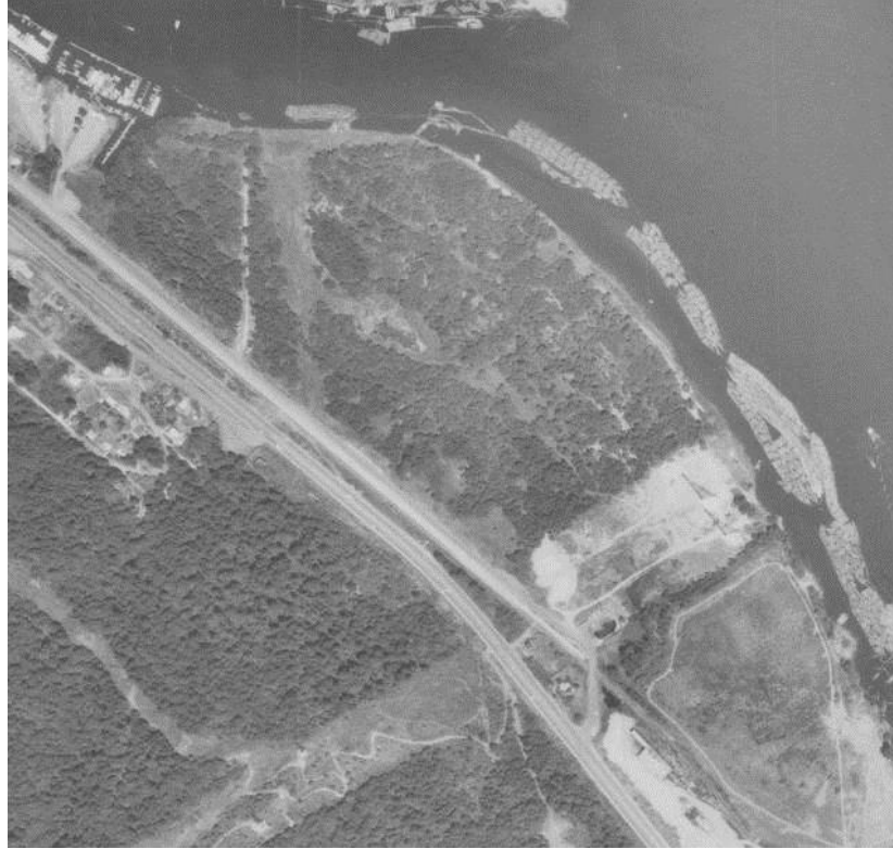
Photograph 3. 1970 aerial photo. Image predates construction of substation. BPA transmission towers, Olympic Pipeline easement, and dike separating Fred's Marina property are evident.
