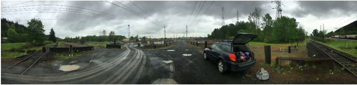
Sub Area 2, panoramic view from access over railroad spur tracks. Taken 4/22/2016
