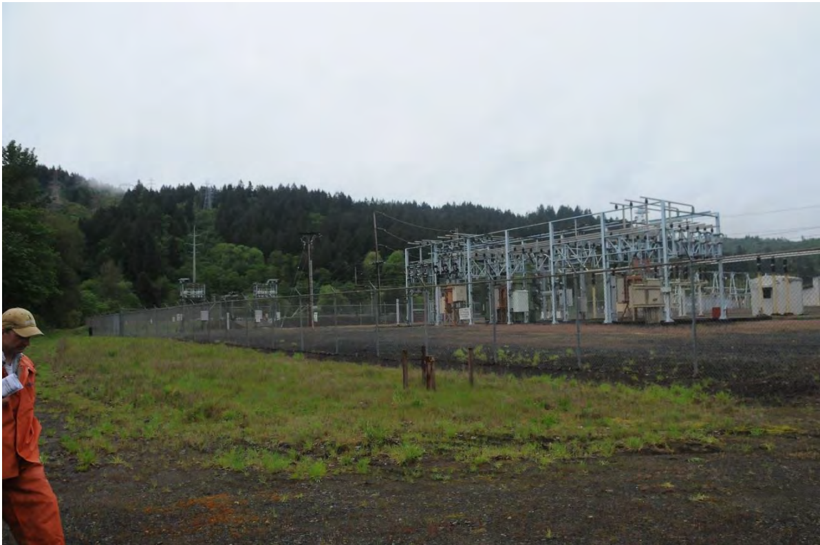
Sub Area 2, existing PGE substation. Taken 4/22/2016
