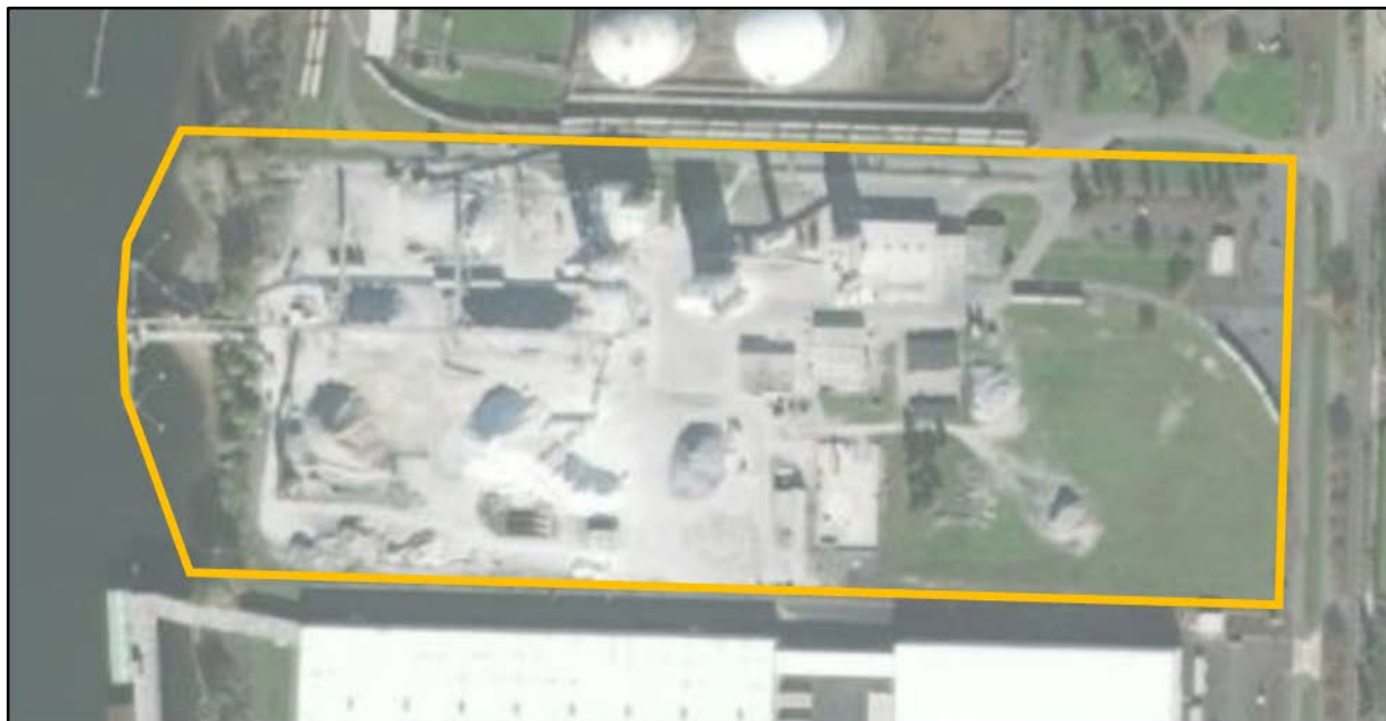
Site 21 – 13939 N. Rivergate Blvd.
